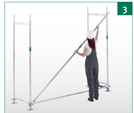
3 Mount diagonal brace on toggle pins.
