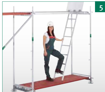
5 Mount inside access deck.
